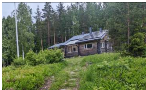
Cottage with solar panels.
